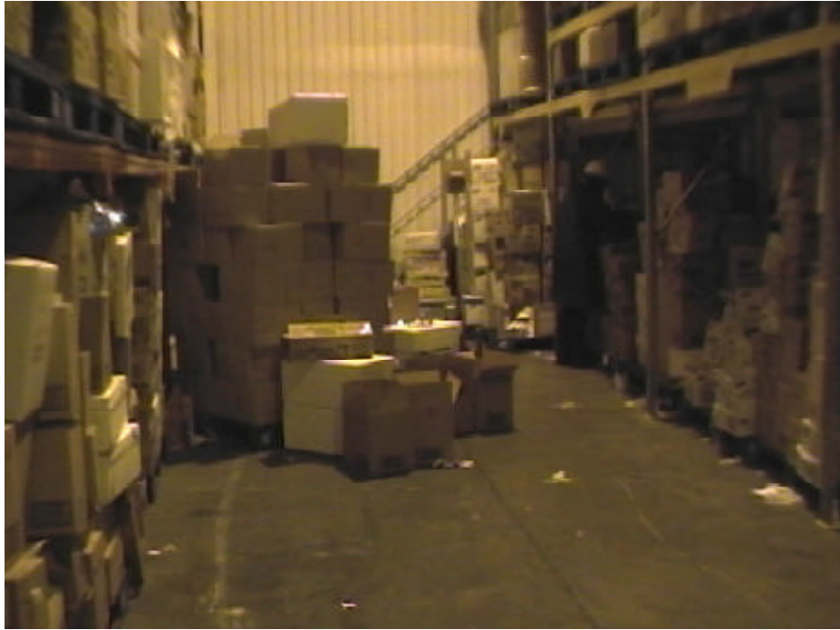
Figure 10: Housekeeping – safe and unsafe situations scored by zone
