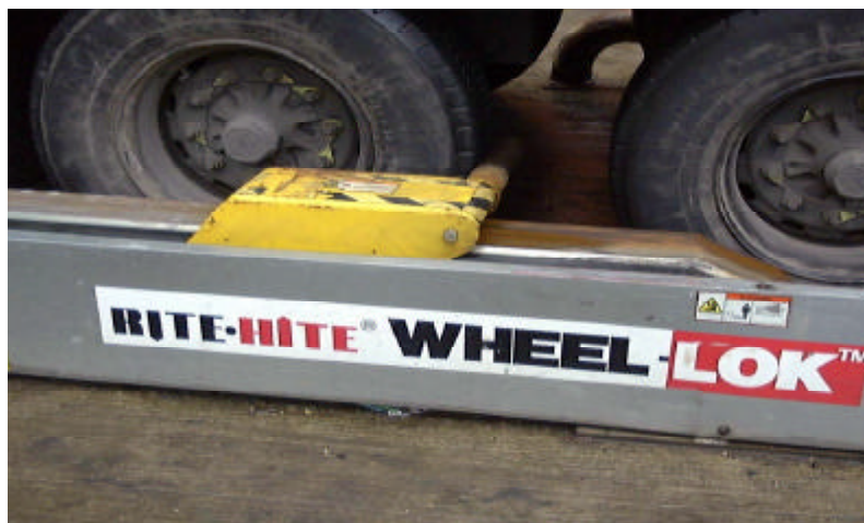
Figure 5.0: Wheel lock to prevent unexpected drive-away of trailers from the Loading Bay area.
