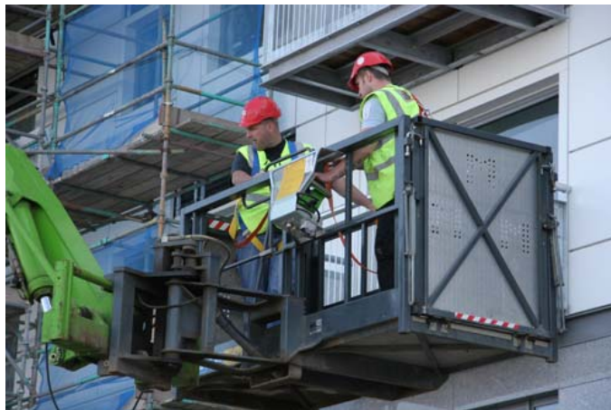
Figure 20 - Integrated Work Platform
